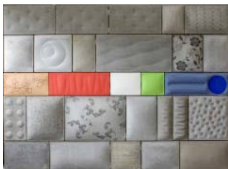
Figure 4 Rain-screen façade using concrete
