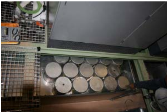
(a) LHS during installation in Spain
