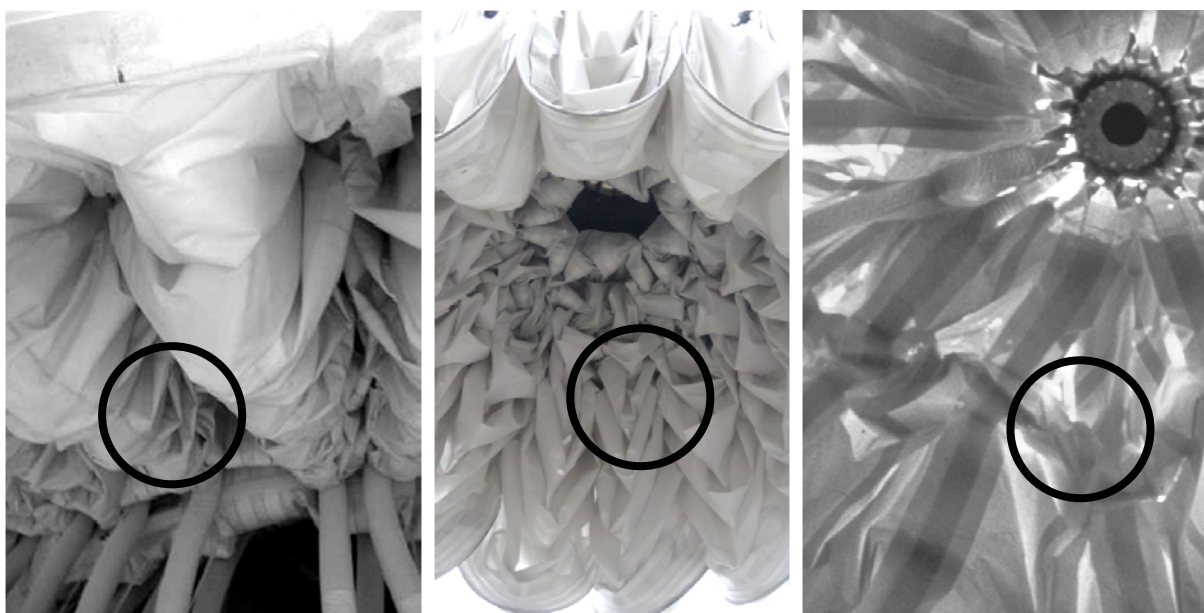
Figure 2: Parked retractable roofs; ruffled to their central point (Kink folds are marked)
