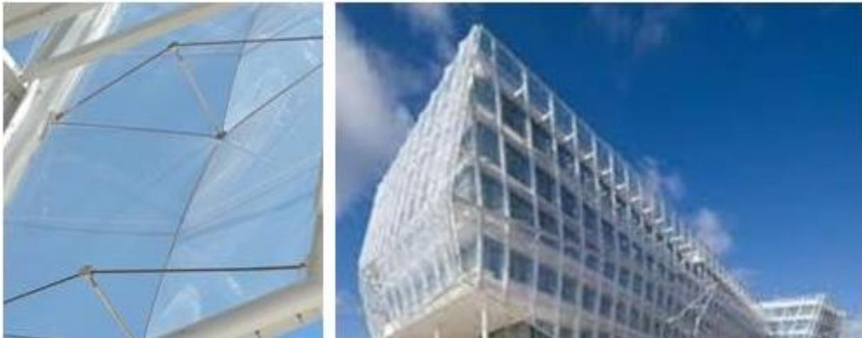
Figure 3: The double curved membrane façades developed for the Unilever building in Hamburg.<sup>6</sup>
