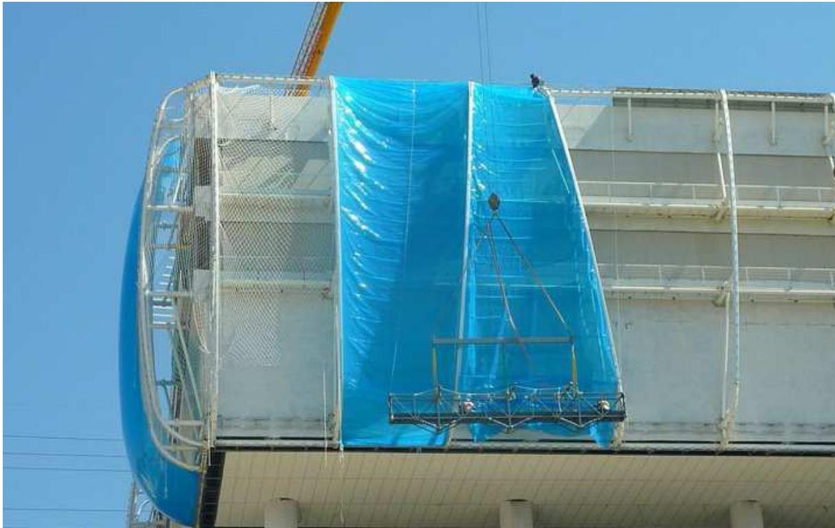
Figure 5: Installation of the Torium Shopping Center pneumatic ETFE façade<sup>8</sup>.
