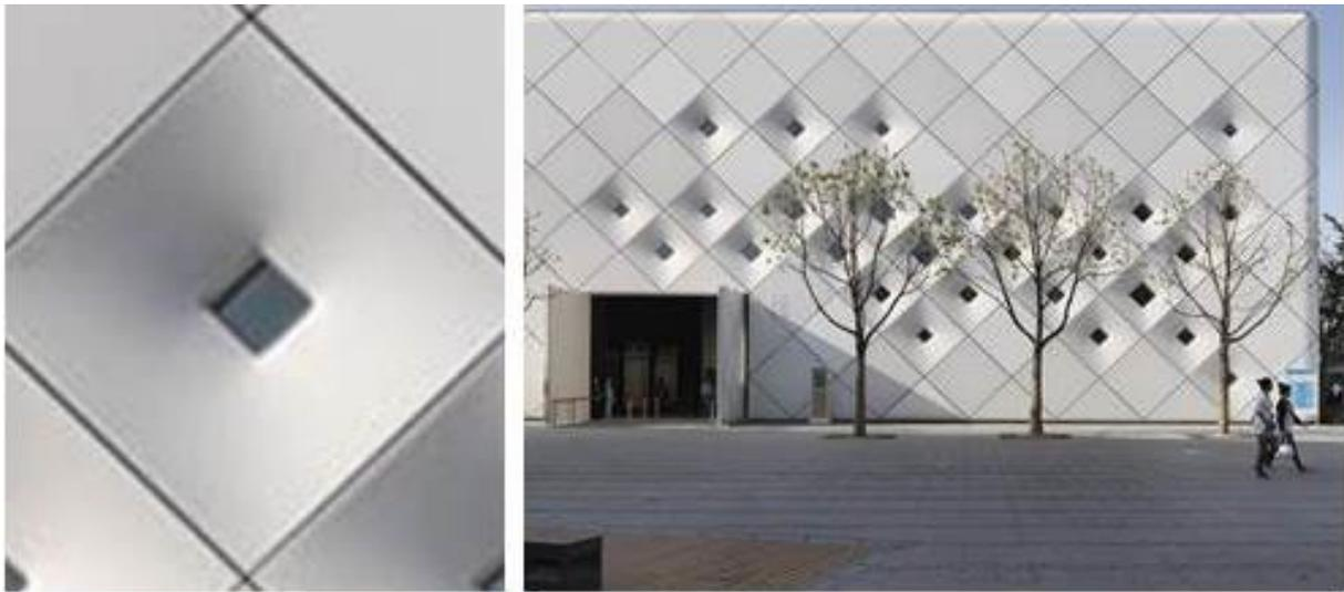
Figure 4: The modular façade for the Expo Shanghai 2010 based on the Texo<sup>®</sup> system<sup>7</sup>.
