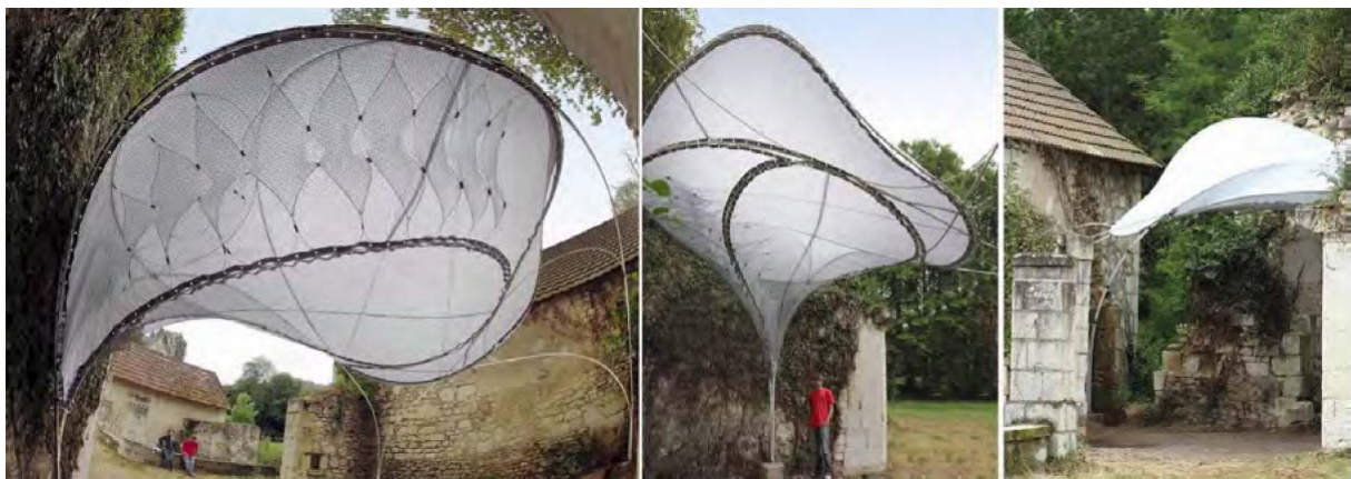
Fig 8: The textile hybrid M1: Internal view of multilayer membrane system with integrated cells. External view in the context of the tower ruin.
