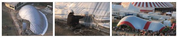
Figure 8: a. Positioning of the PVC coated membrane (Creteil). b. Continuous beam for border during tightening (Creteil). c. Membrane without winkle (Solidays gridshell).
