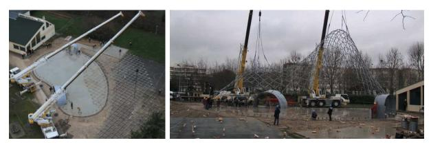
Figure 1. Cathedrale Ephemere de Creteil. a. Primary grid made flat. b. Primary grid deformed elastically and attached to boundary conditions.
