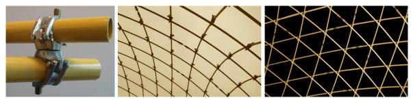
Figure 7: a. Joint detail. b. Mesh before bracing. c. Mesh after bracing.
