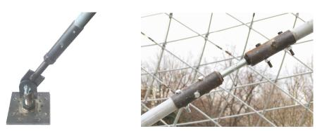
Figure 9: a. Pin anchorage for beams. b. Assembly used to join two beams.
