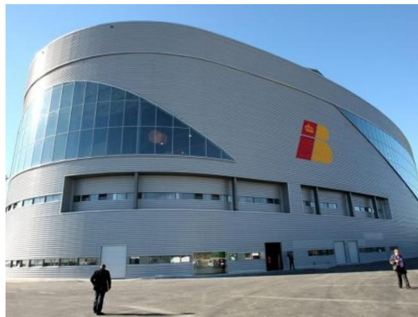
Figure 7.1: Iberia hangar. Source: [5]
