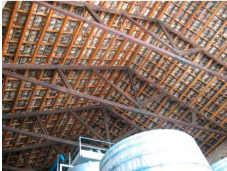
Figure 4. Wood roof trusses in the Falset cellar by Cèsar Martinell, 1919.
