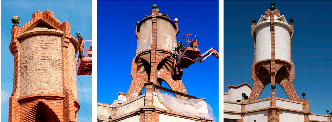
Figure 25. Water tank during restoration ( left and center ). Water tank after restoration ( right ).
