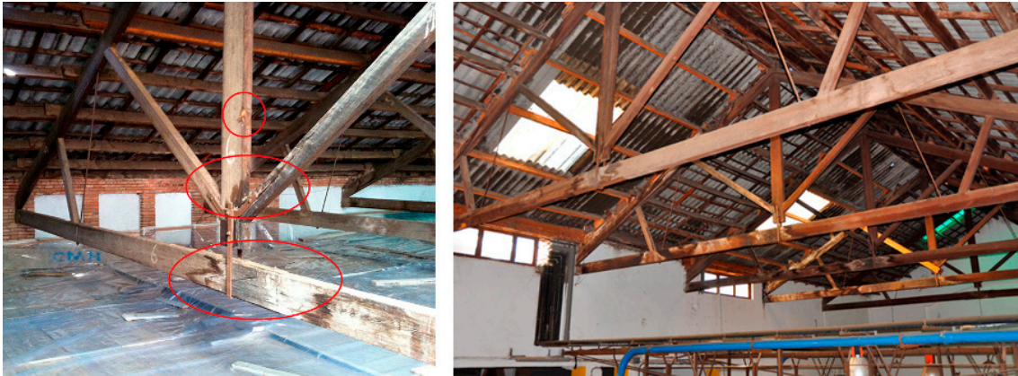
Figure 23. Condition of the production nave roof (interior) before restoration.
