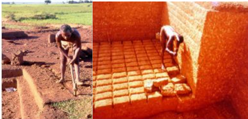
Figure 31: Cutting of sod into blocks [32]
