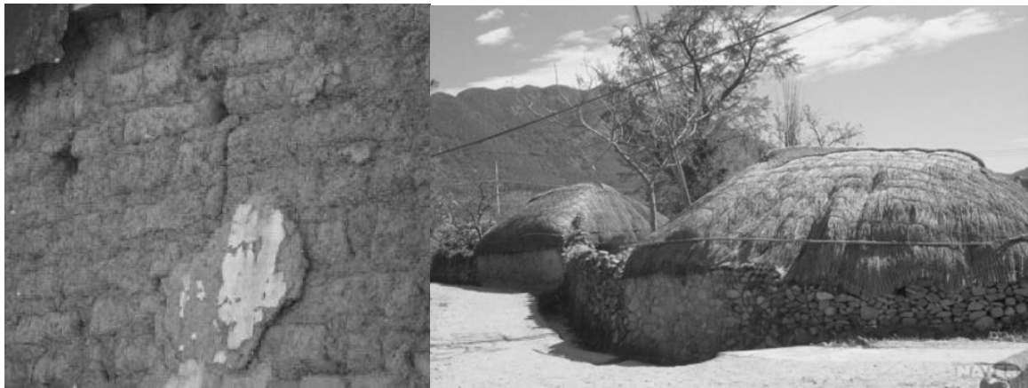
Figure 60: Photograph of earth brick wall of a baracca (left) and a choga (right)
