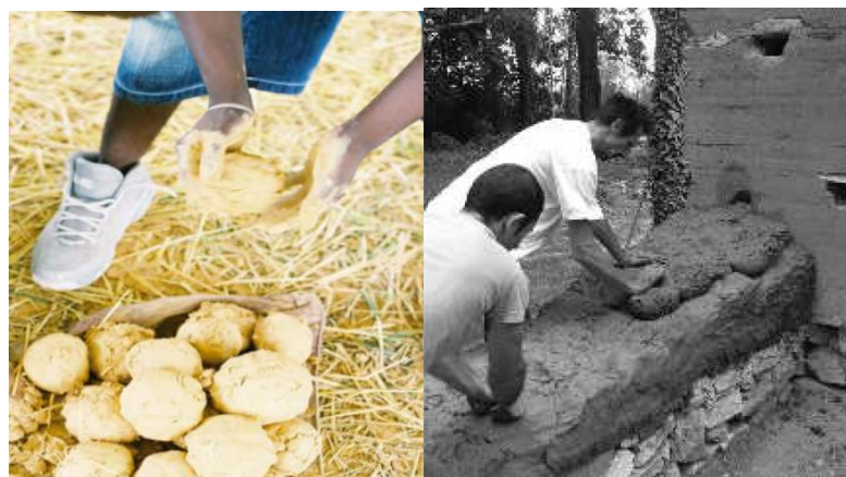
Figure 23: Left: The shaping of a ball [22]; Right: Constructing a cob wall on a masonry base in France [21]
