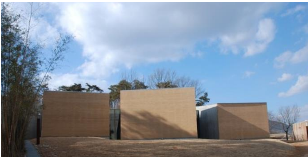
Figure 69: House of Eung-no Lee built part of the exterior walls with rammed earth technique [59]
