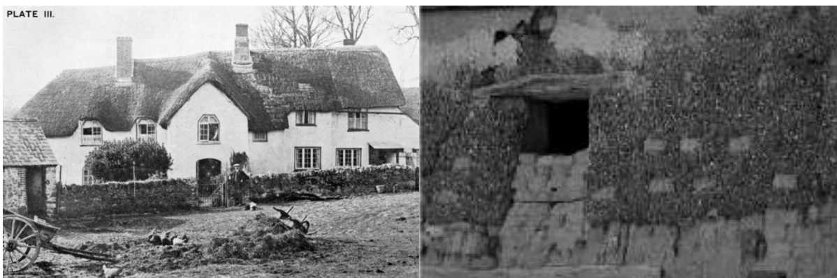
Figure 24: Left: Old Devon Farmhouse from 1920 with cob walls in Devon, UK [23]; Right: Cob wall with adobe reinforcements and a timber lintel in Zamora, Spain [21]
