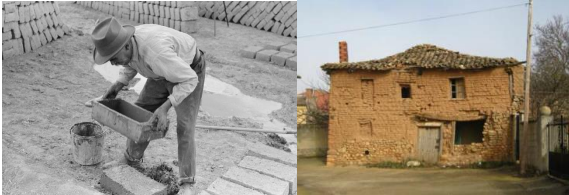
Figure 30: Left: Lifting the mold [30]; Right: Adobe house in Villasandino, Spain [31]
