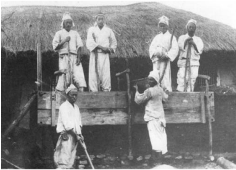
Figure 58: Building a todam with damtle in a typical village in Korea. A photograph is taken by foreign missionaries in the early 20th century.
