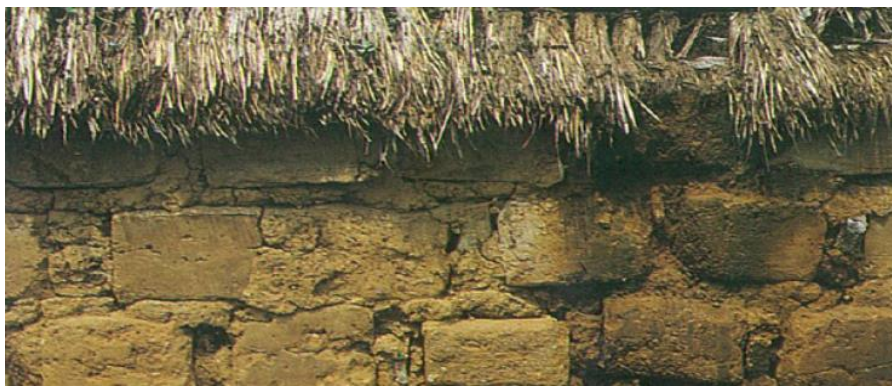
Figure 32: Soil bricks of Fence of Hahoe Village of Korea [33]
