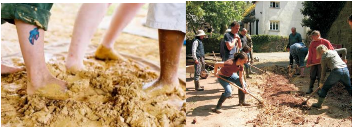
Figure 22: Left: Mixing of subsoil with feet; Right: Adding straws with a shovel in UK [20]
