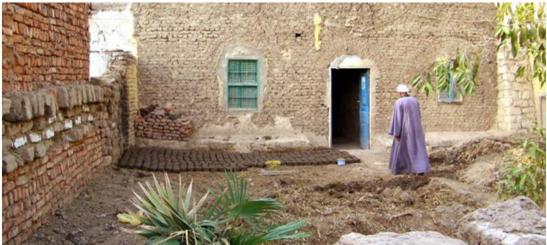
Figure 65: Mudbrick Fabrication in the yard of a Fathy building now under renovation [55]
