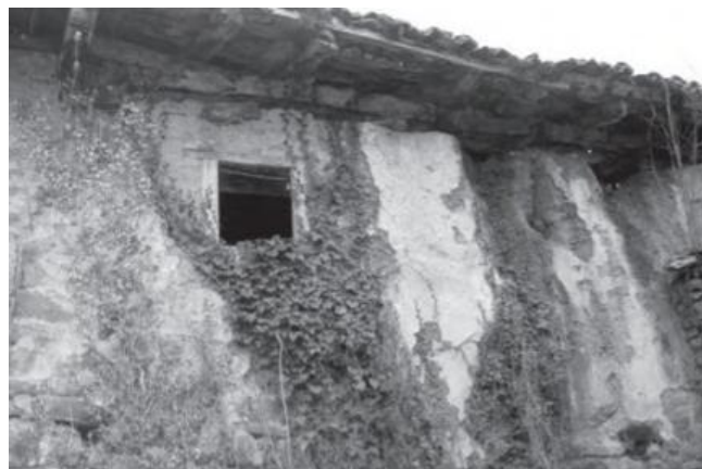
Figure 52: Wall of the barraca built with cob technique [21]
