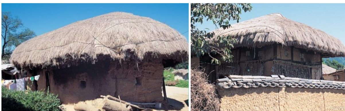
Figure 54: Rammed earth wall (left) and fence (right) of Choga [48]
