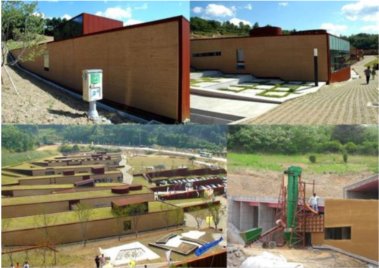
Figure 70: DMZ(Demilitarized zone) Peace Life Park in Korea built with a mix of rammed earth technique, concrete, and corten [59]
