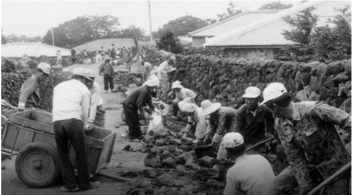
Figure 64: Demolition of earthen buildings in Korea in the 1970s
