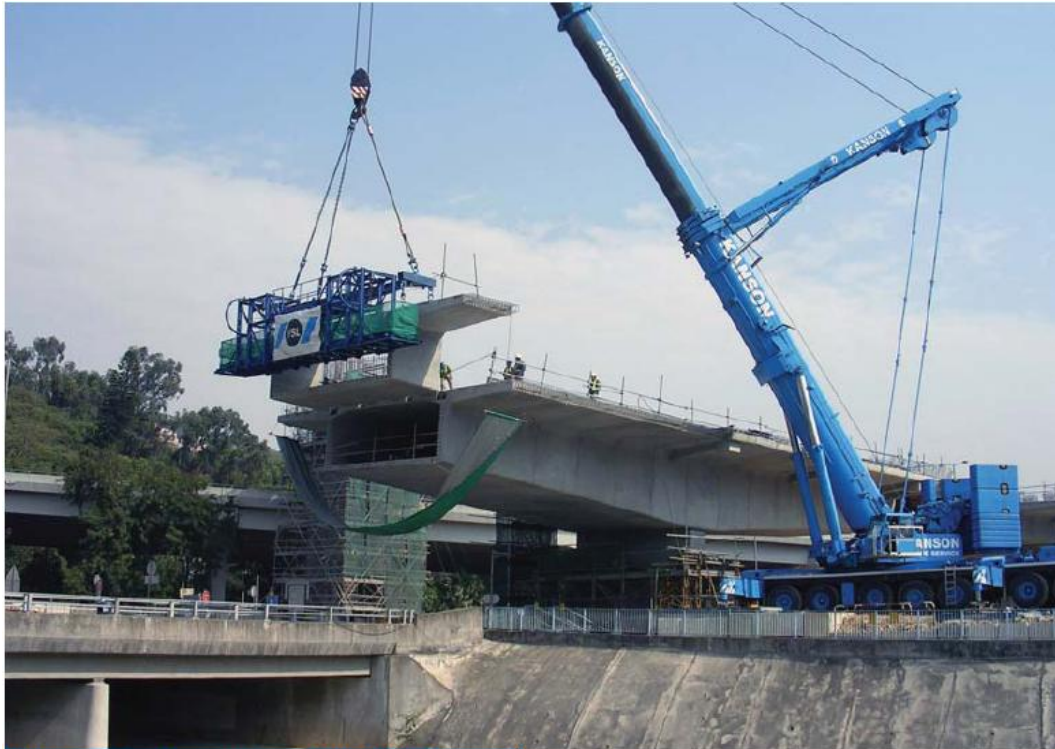
Shatin T3 - Hong Kong (2004-2007) 65,800m 2 of deck, 1,806 segments
