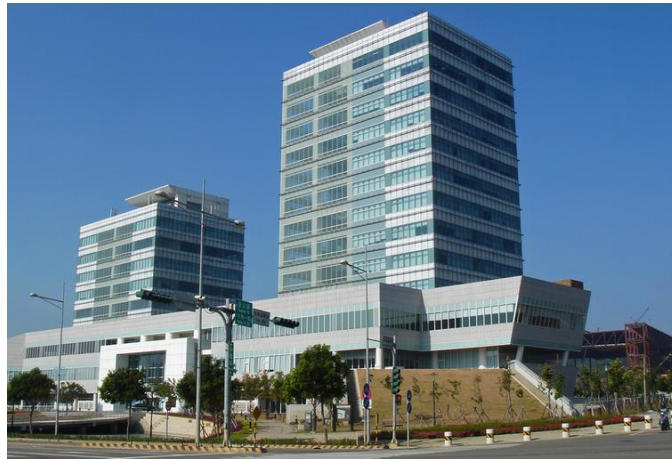
Picture 8. Building studied
