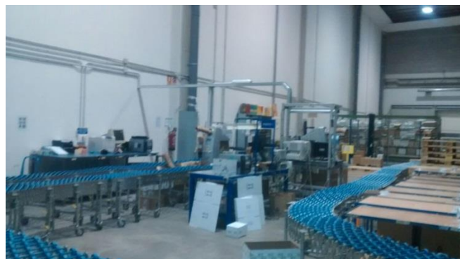
Fig. 3.10.- View of the roller conveyer belts seen from the carousel emplacement. Source [own].
