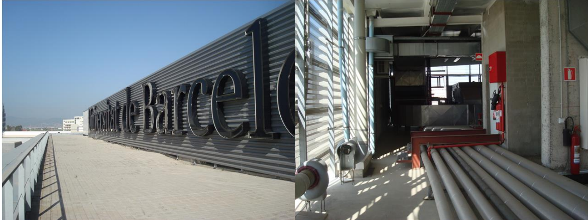
Figure 39: Roof in the fifth floor and TBS area
