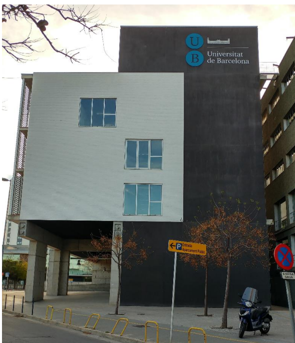
Figure 24: View of the east façade
