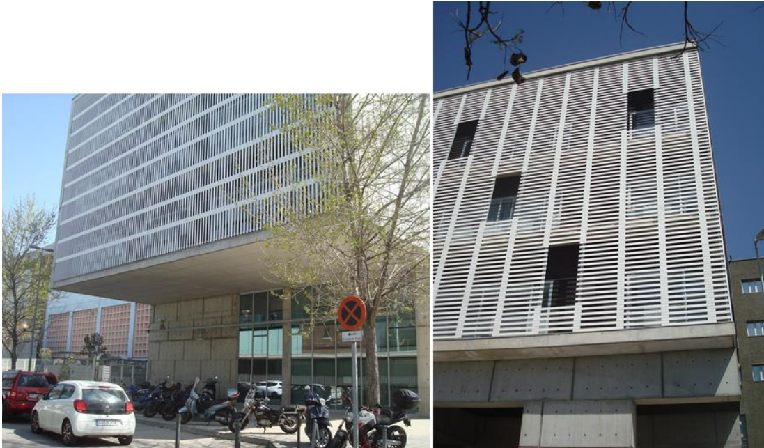
Figure 42: Brise-soleils on west and south-oriented façades
