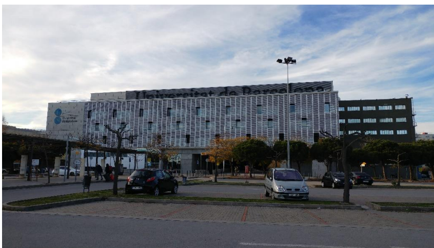
Figure 22: View of the south façade
