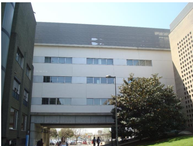
Figure 23: View of the north façade
