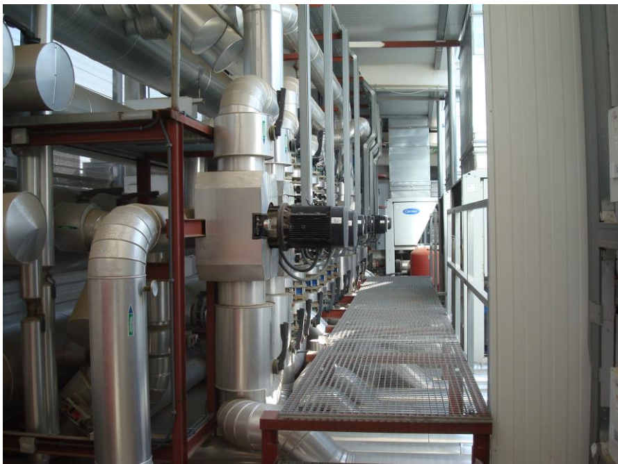
Figure 56: Primary and secondary circuit pumps distribution
