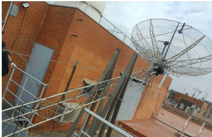
Figure 6.11: Hoisting the antenna
