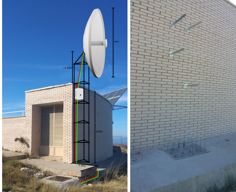
(a) Sketch of the final assembly (b) Foundations laid
