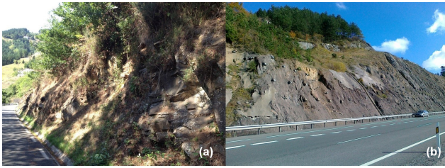
Figure 7. (a) PoR L1C of the road GI-3324 (from km 0.700 to 1.450) without protection measures; (b) PoR P4C of the road N-1 (km 407.395 to 407.680) with protection measures.
