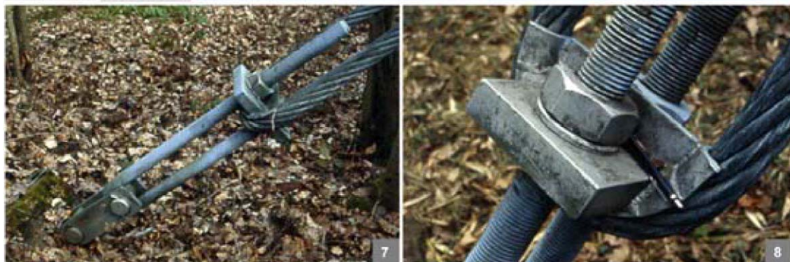
Fittings can also be aggressive or smooth. 1 Aggressiveness is obvious and desired. 2 Cable ends with clips are not smooth. They may cause injuries or damage. 3, 4, 5, 6: Smooth cable ends by Pfeifer: open swaged, turnbuckle with open socket, swaged with thread and closed swaged respectively. 7, 8 The rectangular plate and the cable do not fit together. An adapter is needed. The result looks clumsy.
