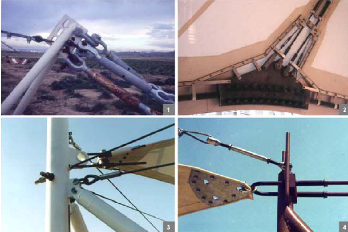
1 Unbalanced situation, three heavy turnbuckles for so little \varnothing 12 mm cable closed with only two clips. 2 Excess of high-tech complexity. 3 Too much everything with different criteria. 4 Different types of fittings look clumsy. In addition, the shackle had to have been long enough to make room for the corner. The cable end is missing the thimble that would not fit in the turnbuckle.
