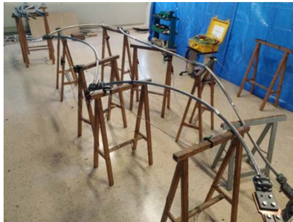
Fig. 3. Temperature rise tests. Test loop composed of HTLS conductors and S285ZTLS T-type mechanical substation connectors.
