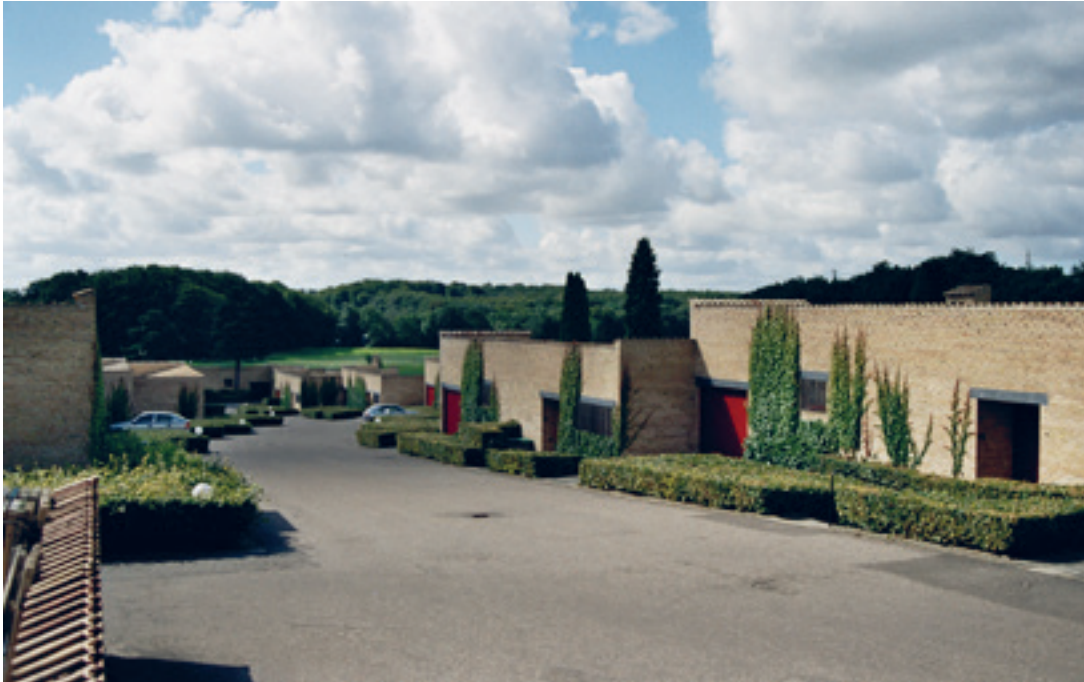
[Fig. 4] Aldo van Eyck. Municipal Orphanage, Amsterdam, 1955-1960. Source: Noelia Cervero Sánchez. Jørn Utzon. Fredensborg patio houses, 1959-1965. Source: Jaime J. Ferrer Forés.
