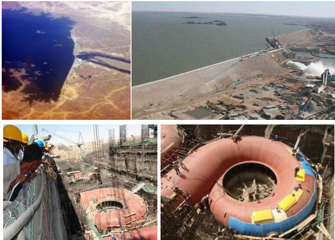
Figure 2 Up: Merowe Dam location and infrastructure 6 . Down: Turbine details 7 .
