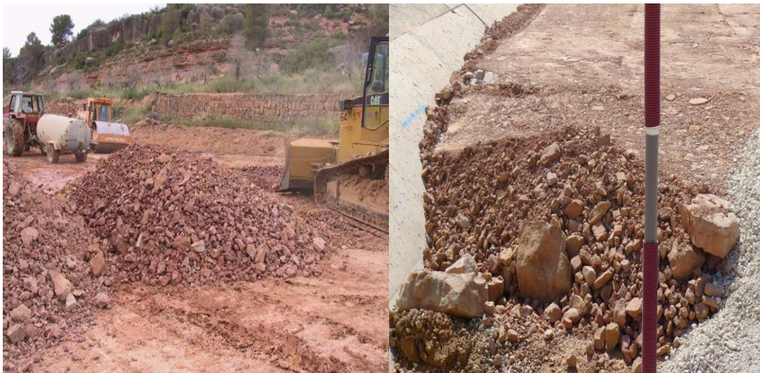
Figure 5-6: The ‘all-one’ material after excavation and during compaction.
