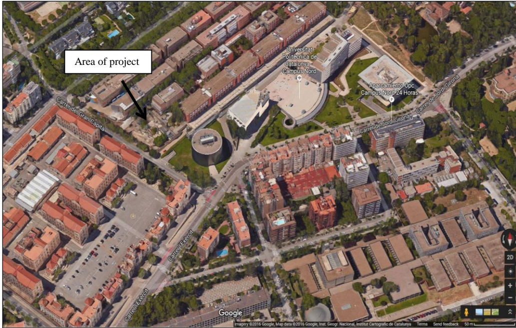
Figure 3-5: Location of building B1project at Universitat Politècnica de Catalunya - UPC campus nord (Google map, 2016).
