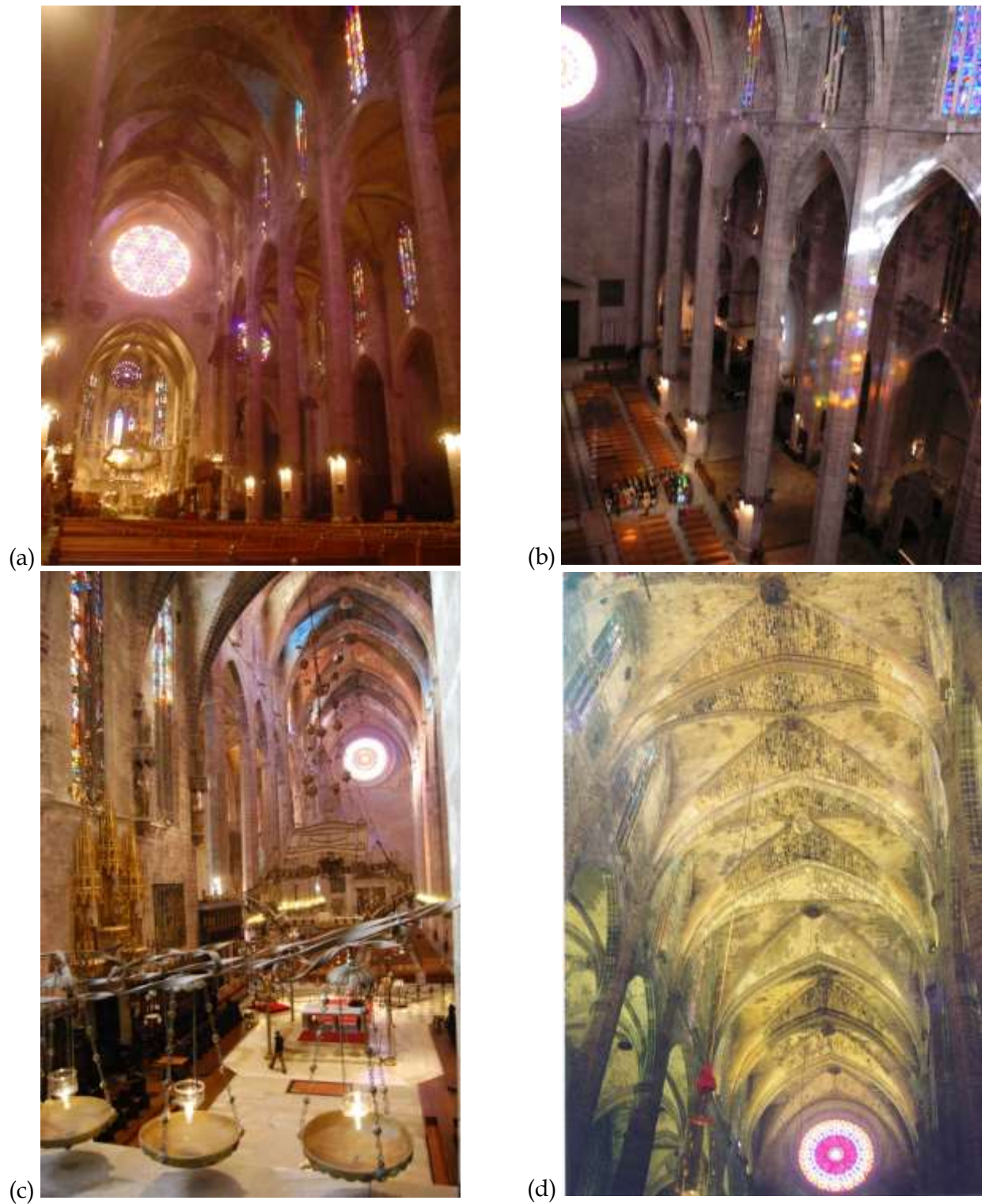
Figure 2. Internal views of Mallorca cathedral: (a) view of the choir, central nave and south lateral nave; (b) view of the west façade and north nave showing the slenderness of columns and the upper and lower clerestory walls; (c) view of the central nave from the choir; and (d) central nave vaults .
