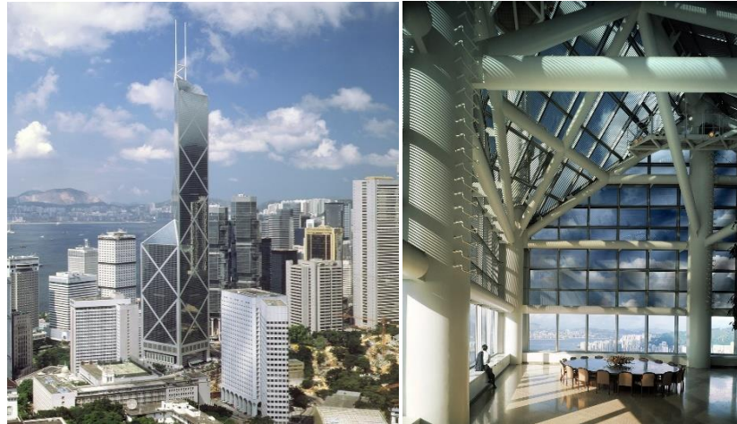
Figure 3: Bank of China tower (Hong Kong)
