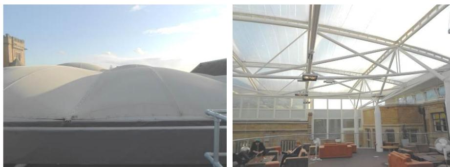
Figure 1: ETFE cushion roof - external (left) and internal (right)
