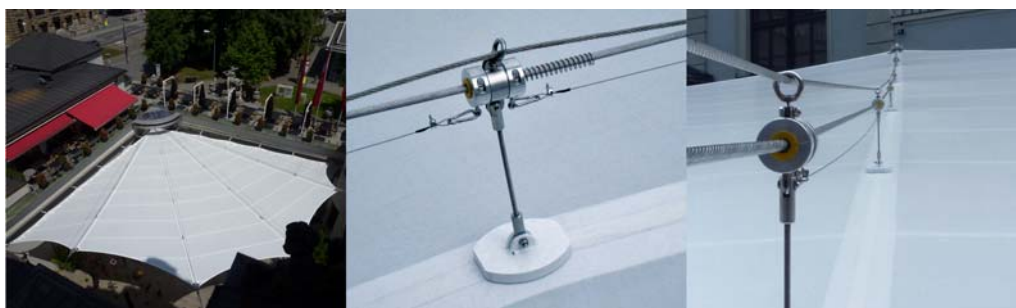
Figure 3: slide bearings with positioning and reef cables
