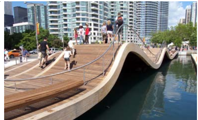
Simcoe WaveDeck and its curves that soar as high as 2.6 metres above the lake.
