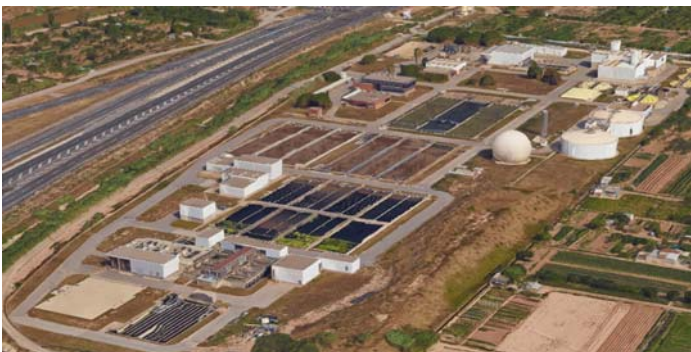
Figure 1: Wastewater treatment plant at San Feliu de Llobregat, Barcelona.
