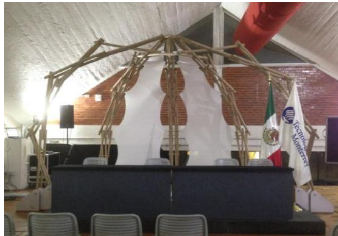
Figure 28. Deployable stage made from cardboard tubing.
