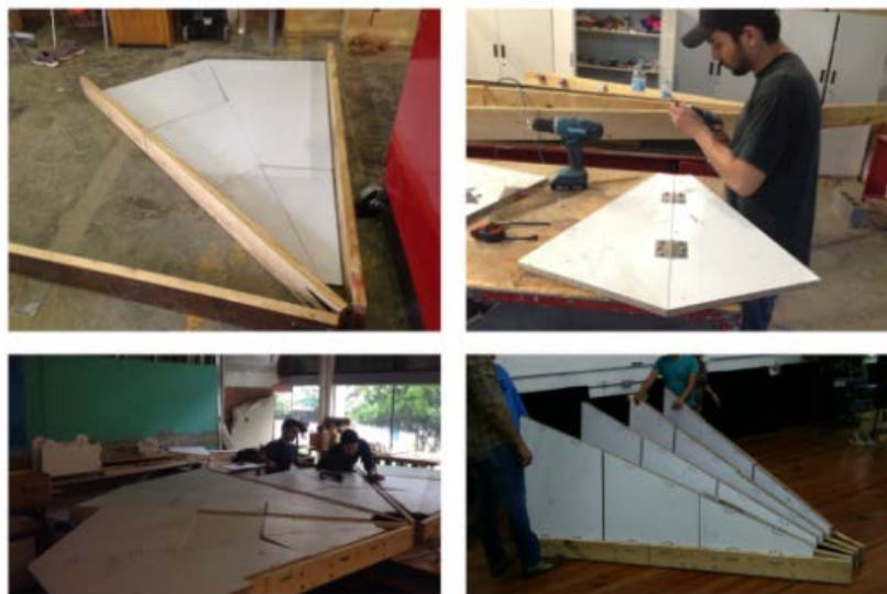
Figure 32. Floor-platform assembly.
