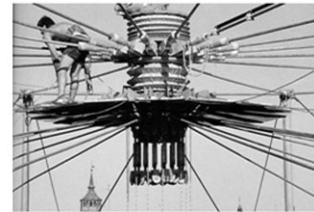
Convertible roof over the Arena, Zaragoza. The central "point" is 3 m in diameter.
