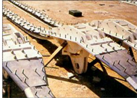
The ridge cables of the cable-dome become strips because the fabric cladding was installed by attaching it to aluminium castings that cover them.
