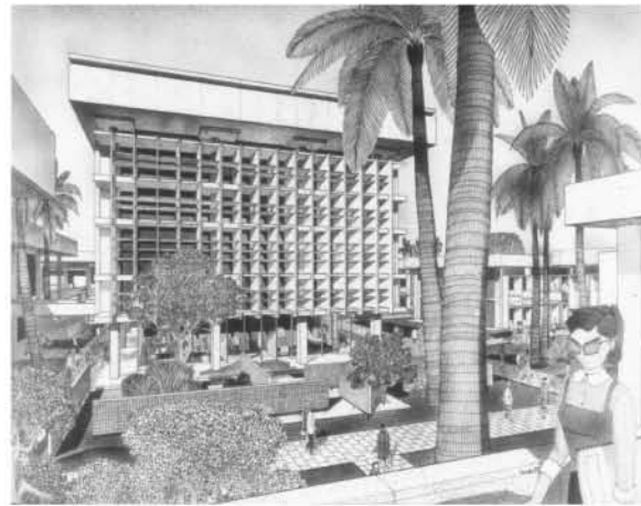
Figure 4. View of the central library from one of the walkways. Sunscreens were an essential design feature for sun protection but, equally important, a prominent sculptural design element Gropius used in all his projects. Using the dikes as walkways allowed different levels and reflect his strict separation of pedestrian and vehicular areas. Drawing by Helmut Jacoby.
