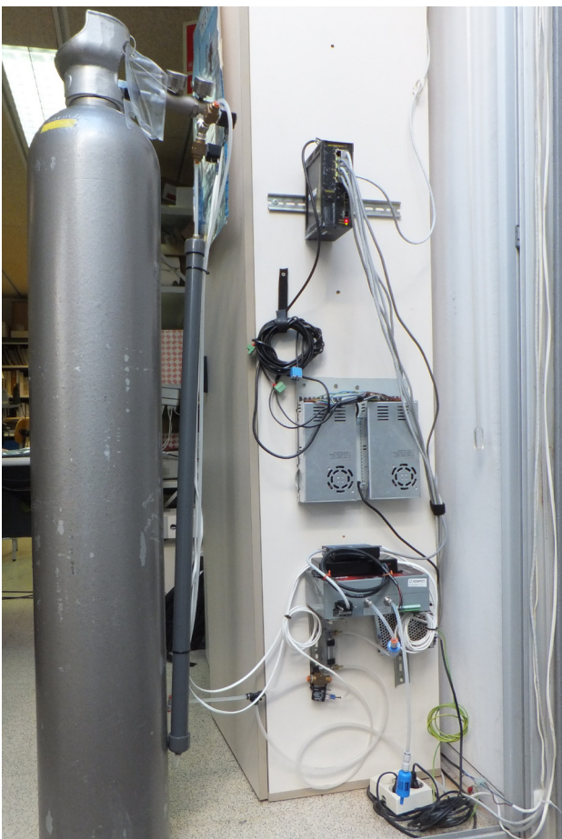
Fig. 3. LI-820 analyzer mounted with the automatic calibration system
