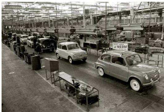
*Fig.1. Manufacture of the Seat 600. July, 1962*
