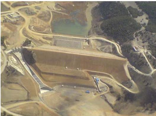
Figure 2: Aerial photograph of Lechago dam at the end of its construction.
