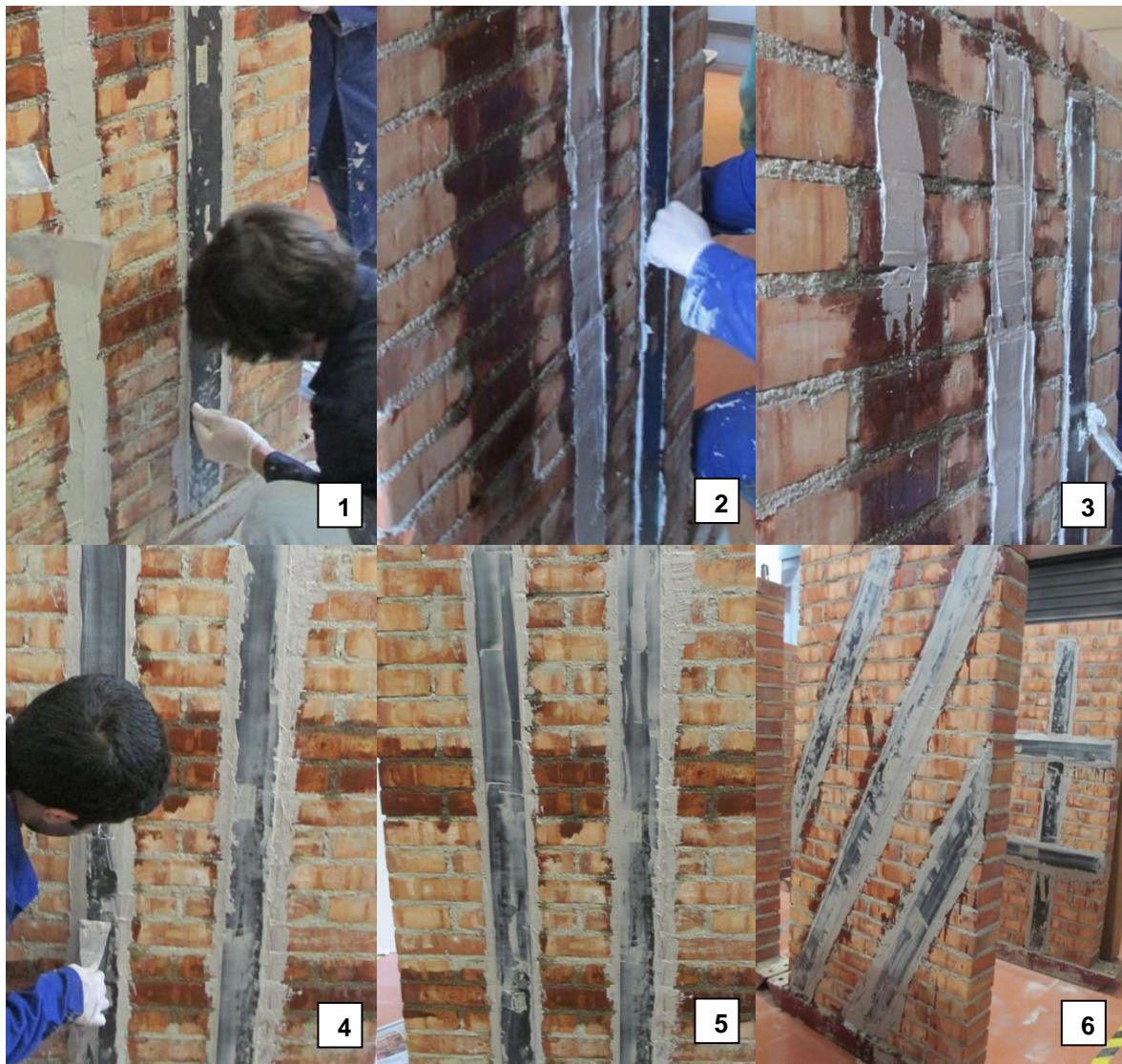
Figure 50 - How to apply the FRPs on walls
