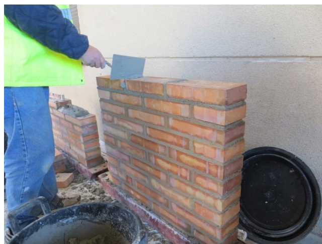
Figure 24 - Process construction of the wall specimens
