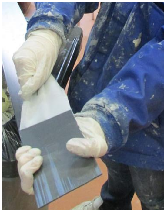
Figure 45 - Removing the protection layer of FRPs for next steps
