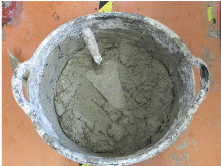
Figure 22 - Preparing the mortar for building the walls
