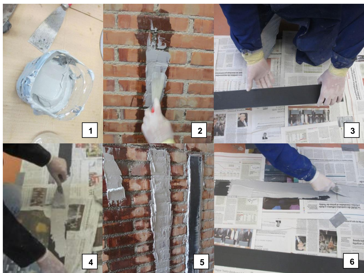
Figure 49 - Process of applying the adhesive on walls and FRPs at the same time
