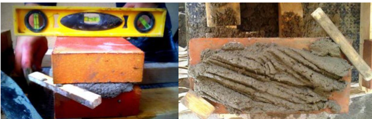
Figure 23 - Controlling the uniform depth of the joints
