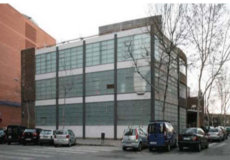
The northern facades and this are made mostly of brick with a few small windows. On the other hand, South and West facades were used glass with metal profiles in most part of this and with a finish of rendering and painted white on the rest of the facade.
