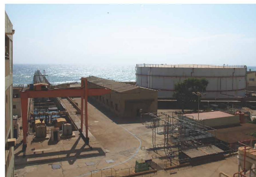
Large fuel tanks
