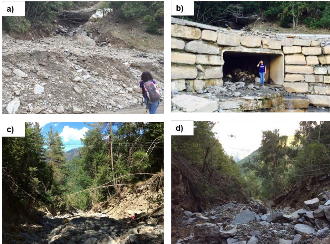
Fig. 5: Field observations of the 2015 debris flow. a) Sediment deposited on the road cross after the 2015 event. Barrier 5 can be observed in the upper part of this photo; b) Obstructed road culvert; c) Section of ultrasonic device before the 2015 debris flow; d) Section of ultrasonic device after the 2015 debris flow.
