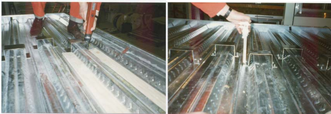
Figure 3.8 Nailed profiled shear connectors
