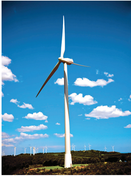
Figure 4.6: ECO-100 wind turbine of Alstom-Wind [2]
