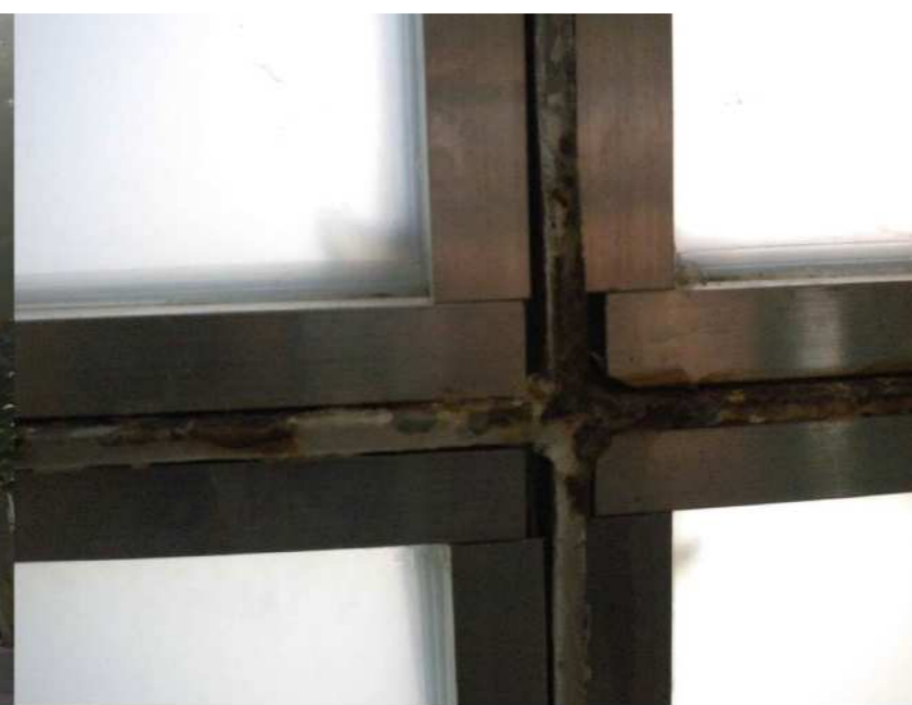
Detall façana principal
