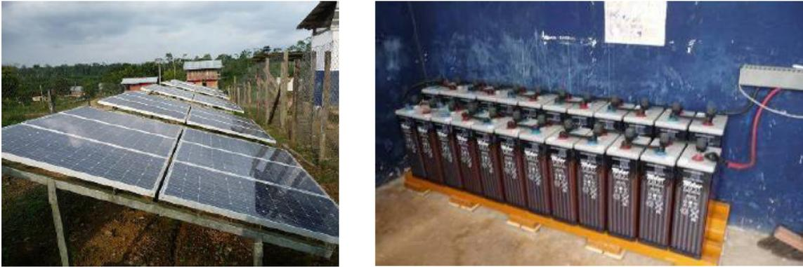
**Figure 2** Stand-alone system: PV generator (left) and battery bank (right). This PV system belongs to a mini-grid located in San Lorenzo, Ecuador.
