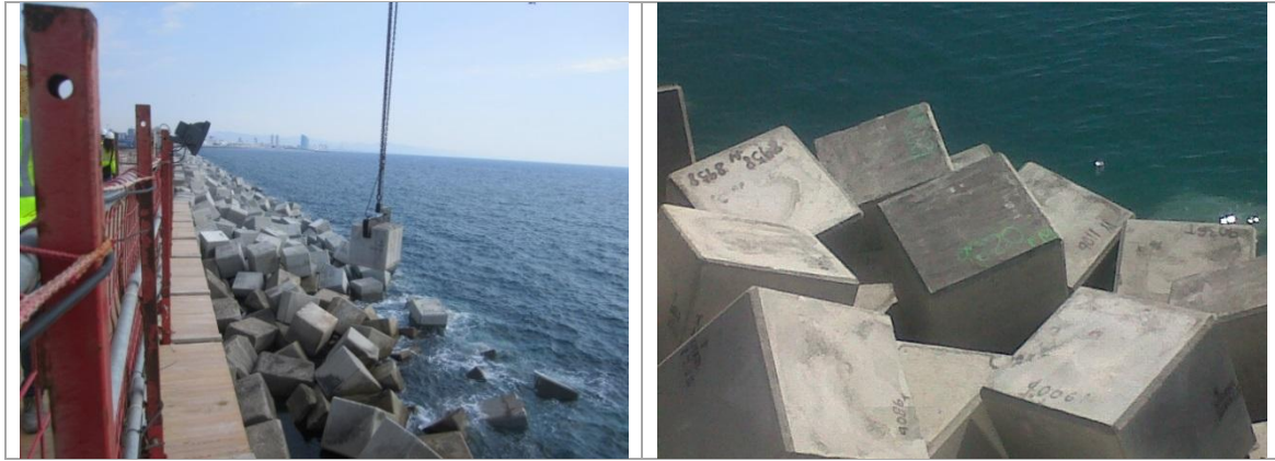
Figure 2. Production process and placing of concrete blocks
