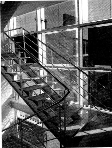
Figure 10. Interior of staircase.
