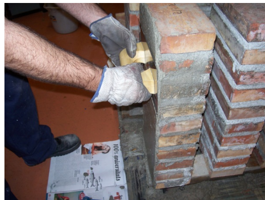
b) Applying the first mortar layer
