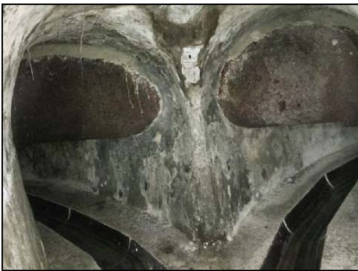
Fig. 4. Section reduction by transversal pipes.
