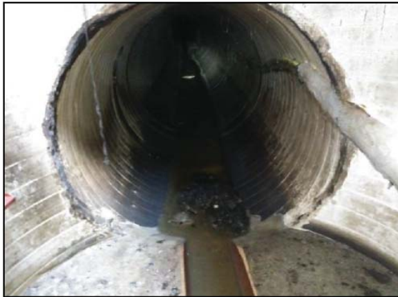
Fig. 3. Connections between pipes.
