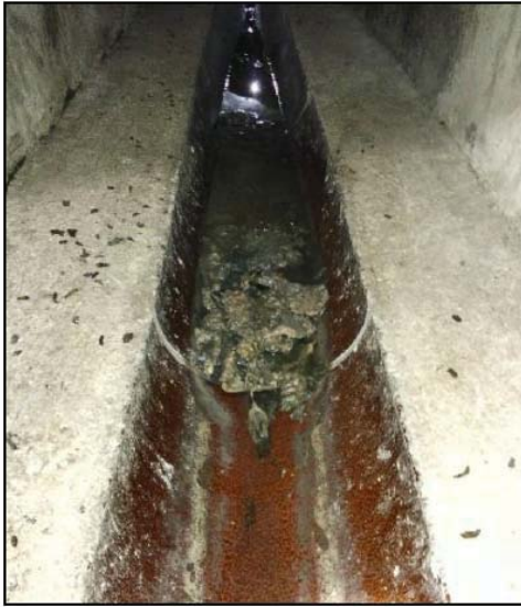
Fig. 2. Sewer obstruction.
