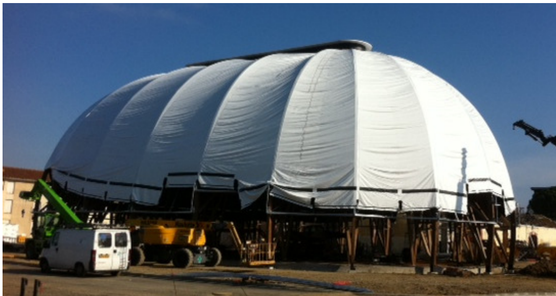
Figure 8 : View of the first layer of membrane
