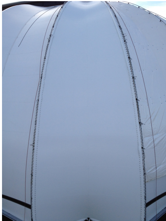
Figure 12 : Three layers are visible: Left inner membrane, Right isolation layer, Centre outer membrane
