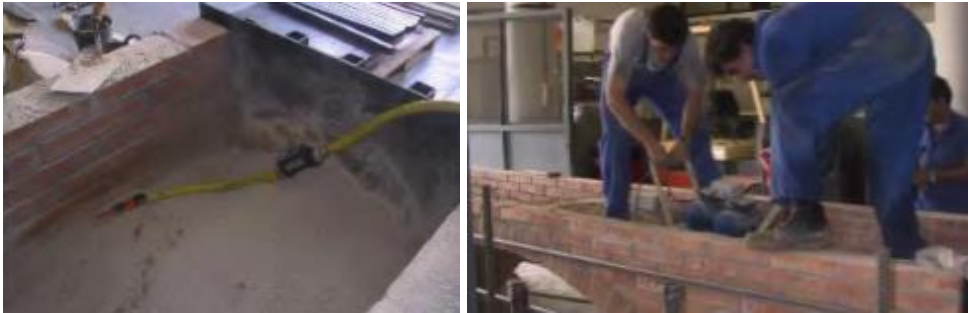
Figure 3-9 filling and compacting of the infill (Serna, J., 2001).
