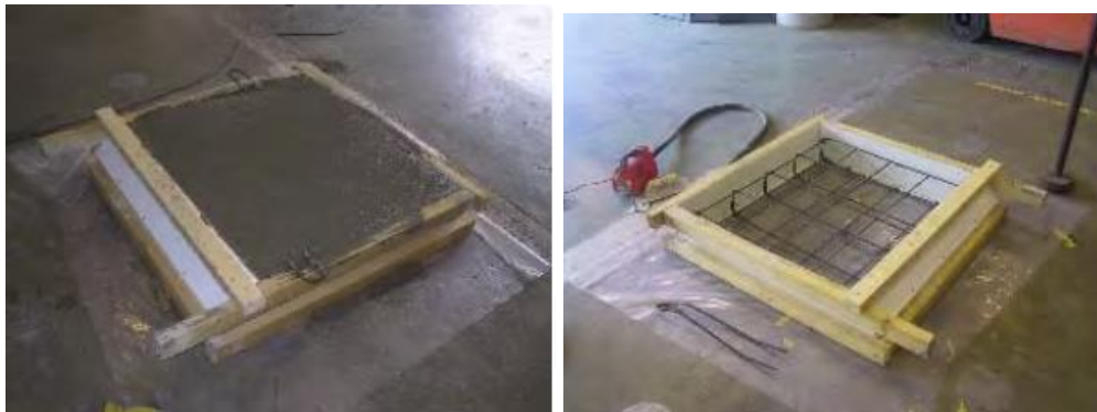
Figure 3-5 formwork and concreting of the slabs (Serna, J., 2001).
