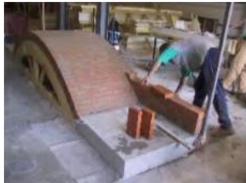
Figure 3-7 construction of ring and spandrel walls (Serna, J., 2001).
