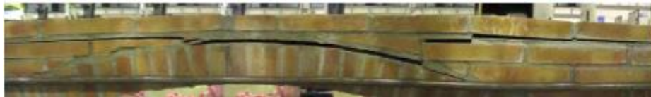
Figure 3-22 view of the two plastic hinges in the east side (Serna, J., 2001).
