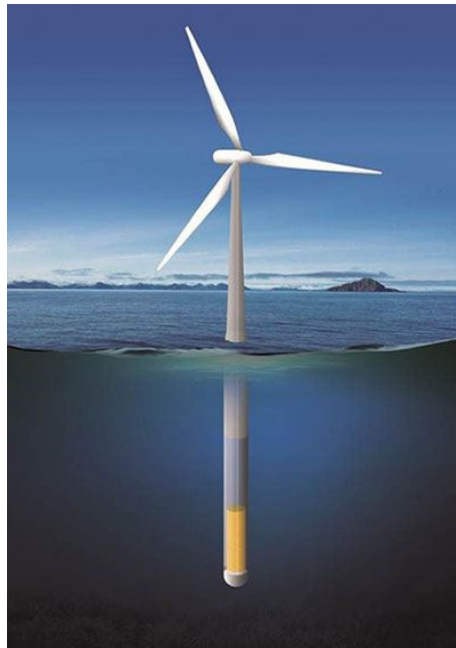
Figure 4 3D render of the WindCrete conceptual concrete structure for floating wind turbines.
