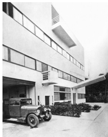
Figure 4. Le Corbusier. Les Terrasses , Stein house, Garches, near Paris, 1927-28 (Modern Architecture: International Exhibition, 1932).
