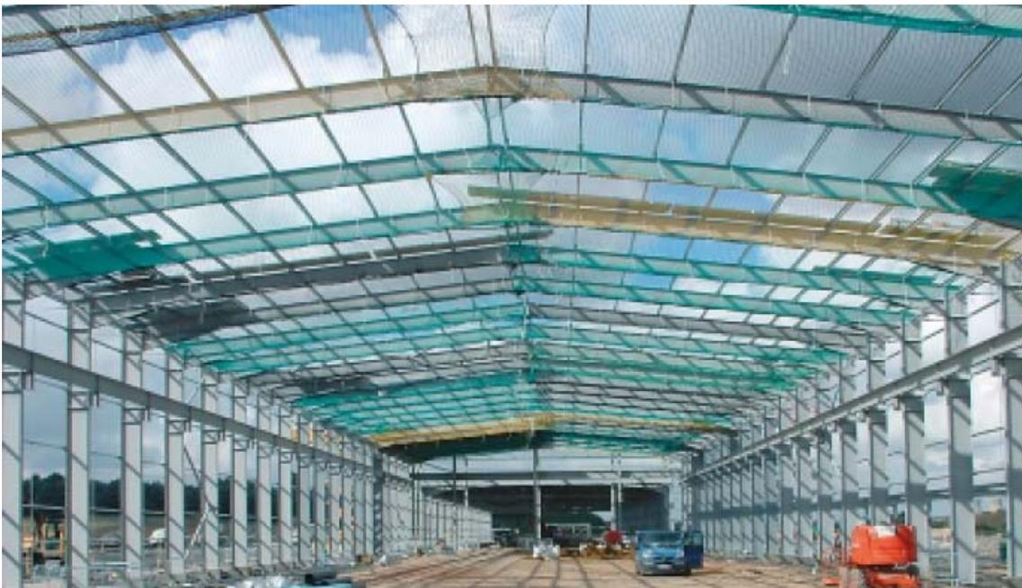
*Fig 1.15: Framed building with purlins, before laying the roof and walls. Extracted from [11]*
