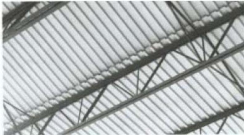
*Fig 1.14: Metal sheets laid on a bar joist frame. Extracted from [9]*
