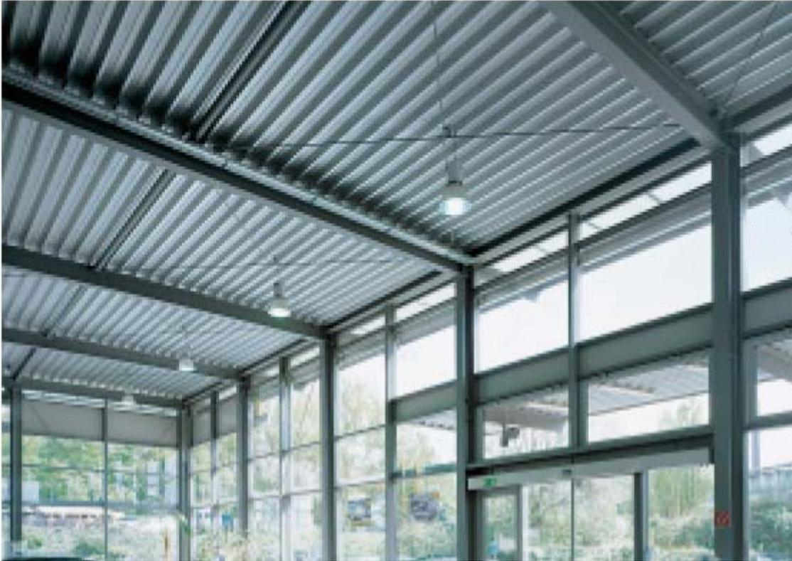
*Fig 1.15: Metal sheets laid on a the rafters Extracted from [10]*
