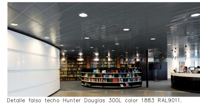
Detalle falso techo Hunter Douglas 300L, color 1883 RAL9011.
